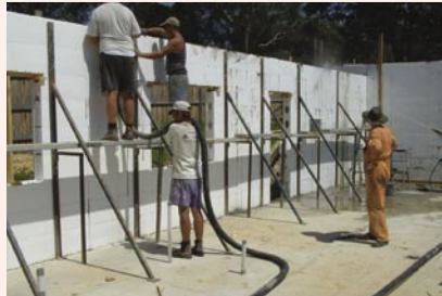
To wall construction
